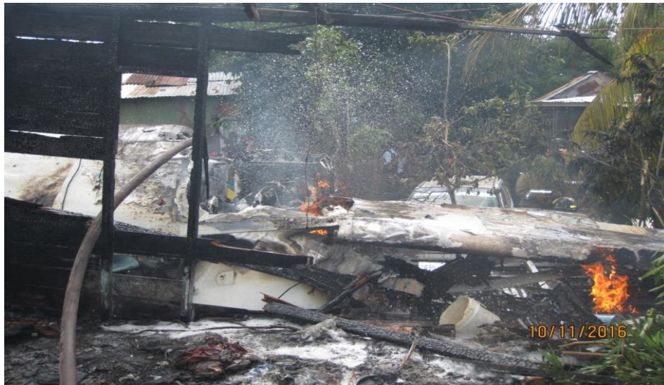
Figure 27 Fire Damage to the Aircraft Fuselage
