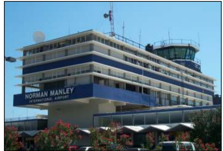
Control Tower at the Norman Manley International Airport (NMIA) Port Royal Road Kingston
